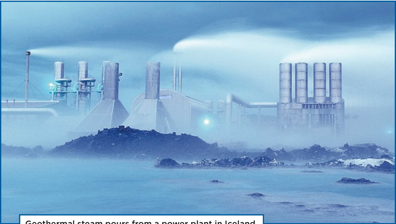
Geothermal steam pours from a power plant in Iceland.
