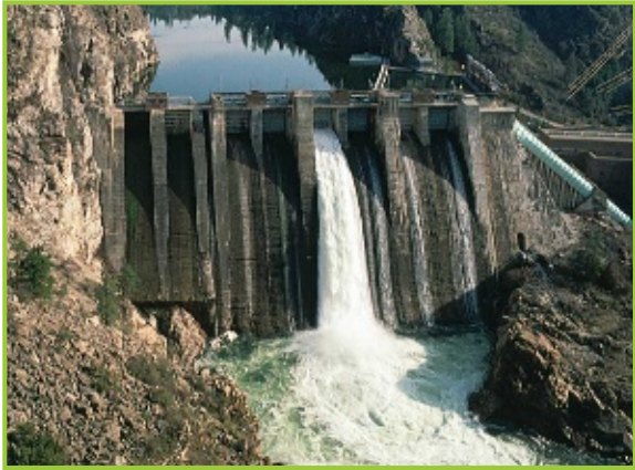
▲ A dam collects and stores the water that will be used to run a hydroelectric power plant's turbines.
