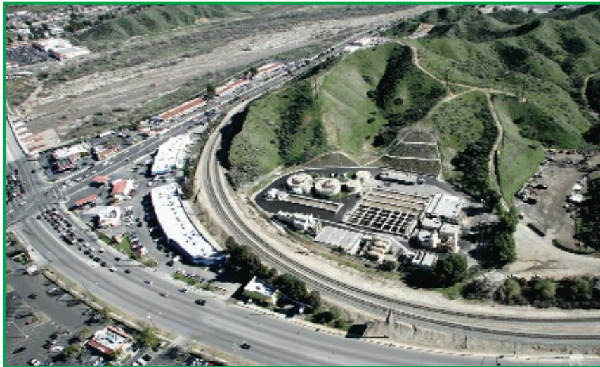
The Sangus Water Reclamation Plant in Santa Clarita cleans 7 million gallons of used water each day.
